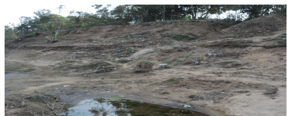
Embankment in Subarnarekha River not restored
